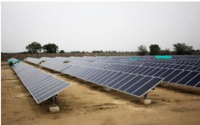
Tracker System (ground mount) (NBC Bearings, Jaipur, 443 kWp)
