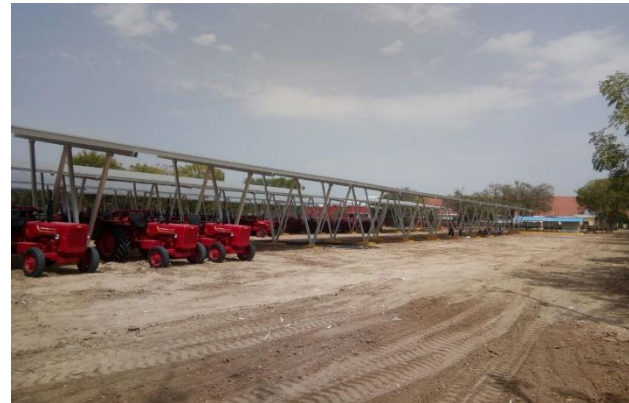
Tractor Parking Structure with metal sheet (Mahindra Tractors - Jaipur)
