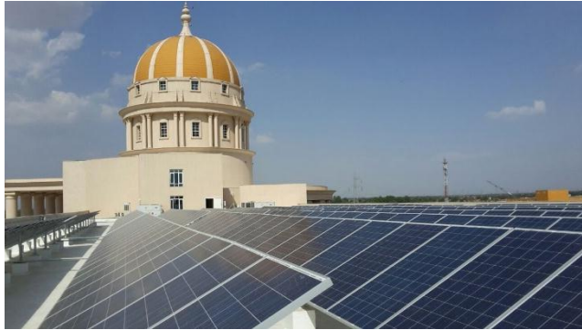
RCC Installation (Manipal, Jaipur, 1 MWp)
