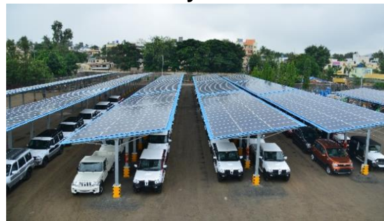
Carport Structure with metal sheet (Mahindra & Mahindra – Nashik)
