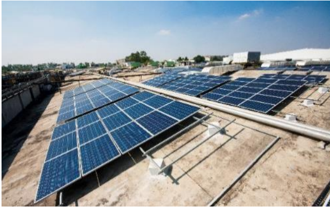
Sloped RCC Installation (SKF India, Bangalore, 1 MWp)
