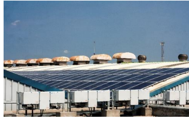
Curved Metal Roof Installation (Asahi Glass, Chennai, 2.6 MWp)
