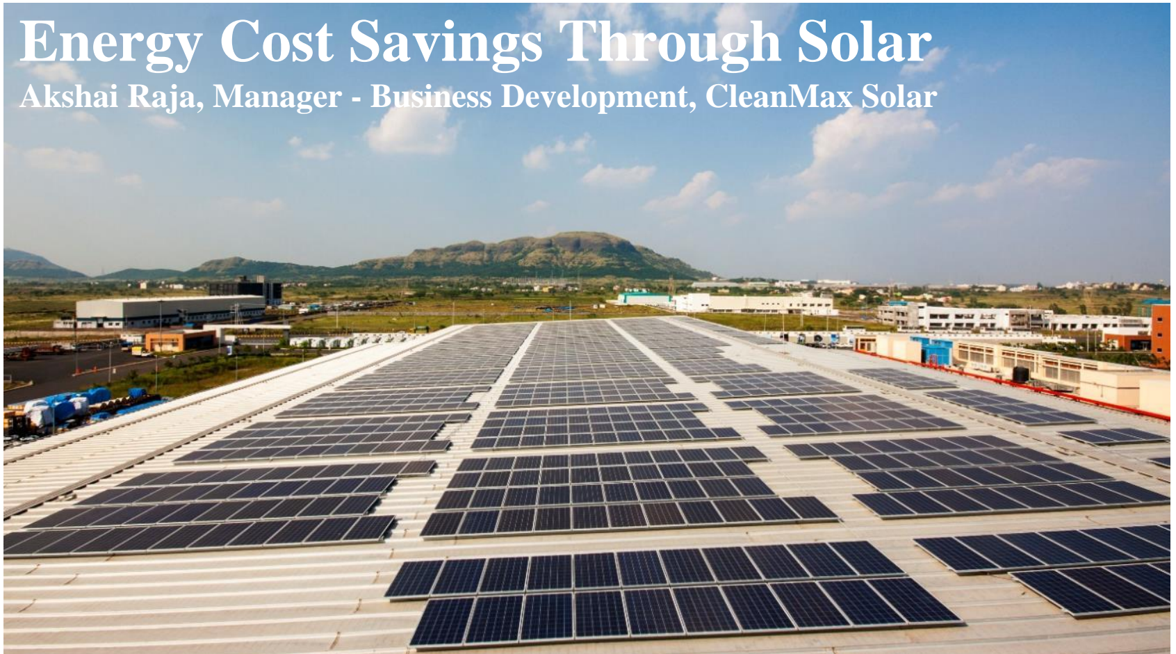
CleanMax Rooftop Solar Installation at leading MNC in Pune, 550 kWp
